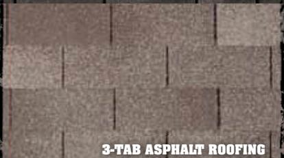
3-TAB ASPHALT ROOFING
